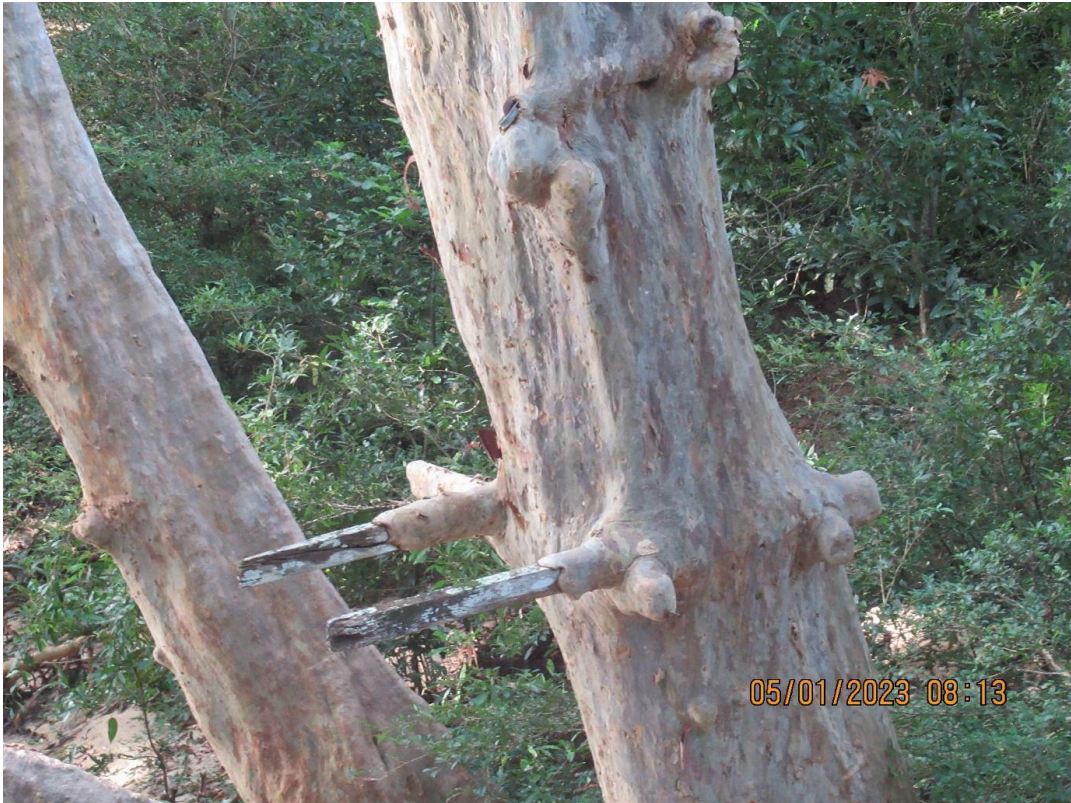
Figure 33. The remains of the old suspension bridge embedded in the tree. (Photo by C. Mendis, 2023).
