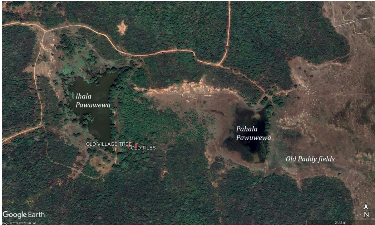
Figure 28. Location of the roof tiles of the abandoned village between the two tanks (Google Earth imagery, 2024).
