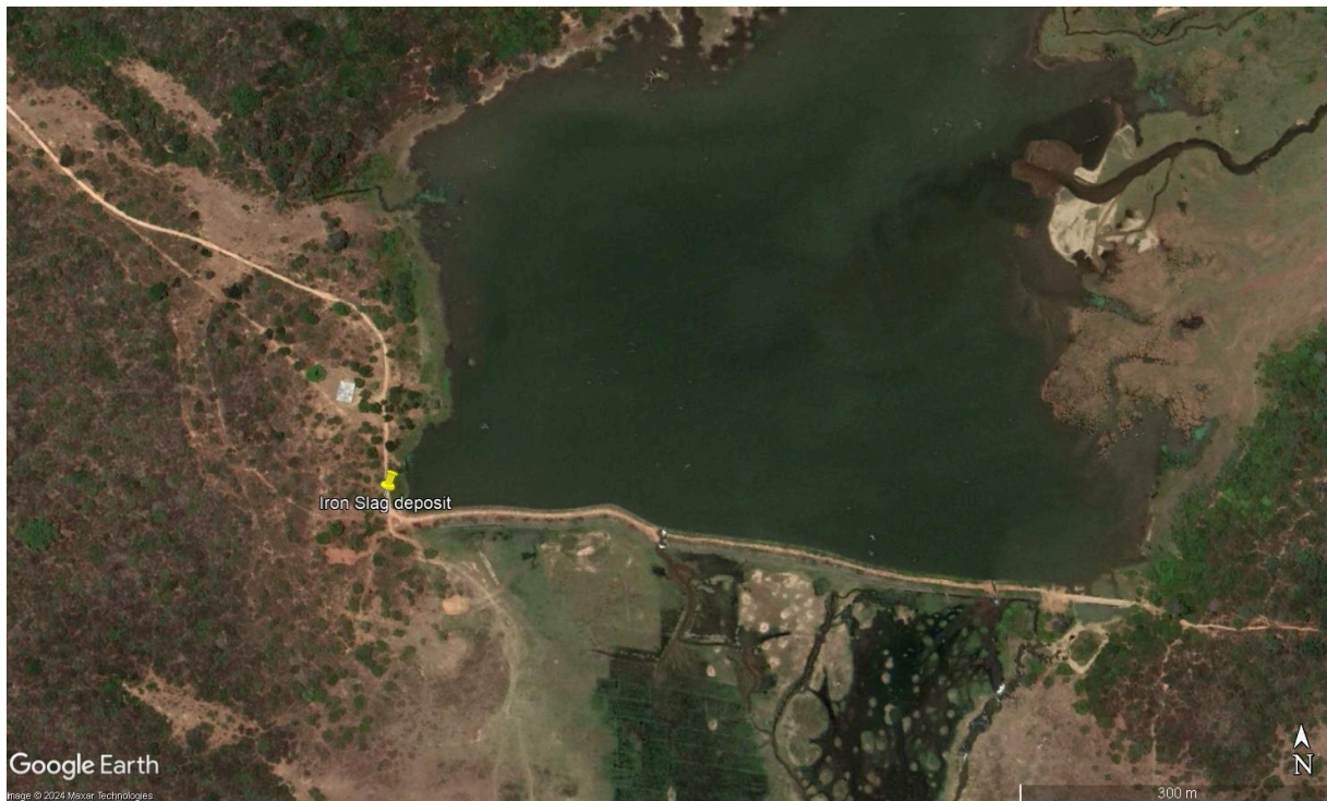
Figure 36. The Rathmal Wewa with iron slag deposit. The traces of old paddy fields can be seen here below the bund. (Google Earth imagery, 2024).
